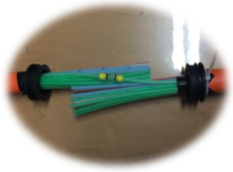
Connect microtubes outside of closure.
