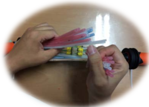
Connect microtubes starting from inside to outside ones.
