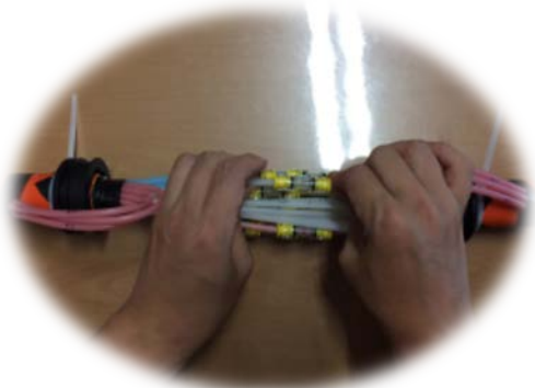
Connect microtubes starting from inside to outside ones. (2)
