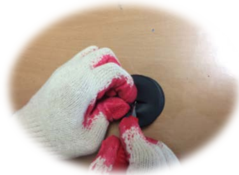
Make a hole of rubber sealing cap to fix the microduct.
